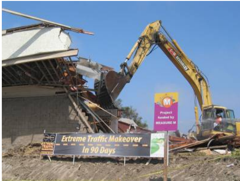
Demolition event for 90-day traffic makeover
