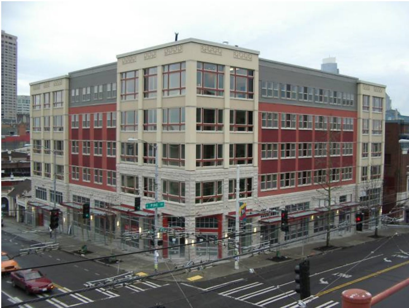
Seattle, WA – Broadway Crossing
