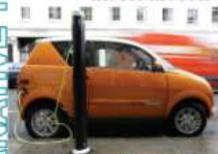
ELECTRIC VEHICLE CHARGING STATIONS
